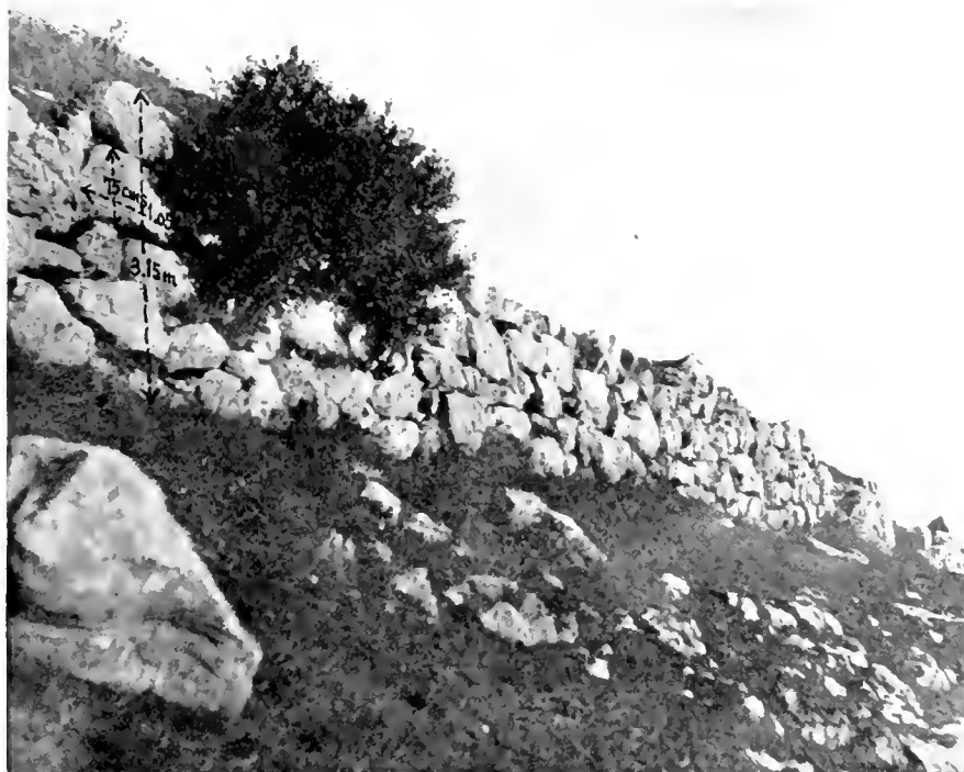
FIGURE 4. — A PIECE OF THE OUTER WALL ON THE WEST SIDE Near point A, between the posterns at Nos. 6 and 7
